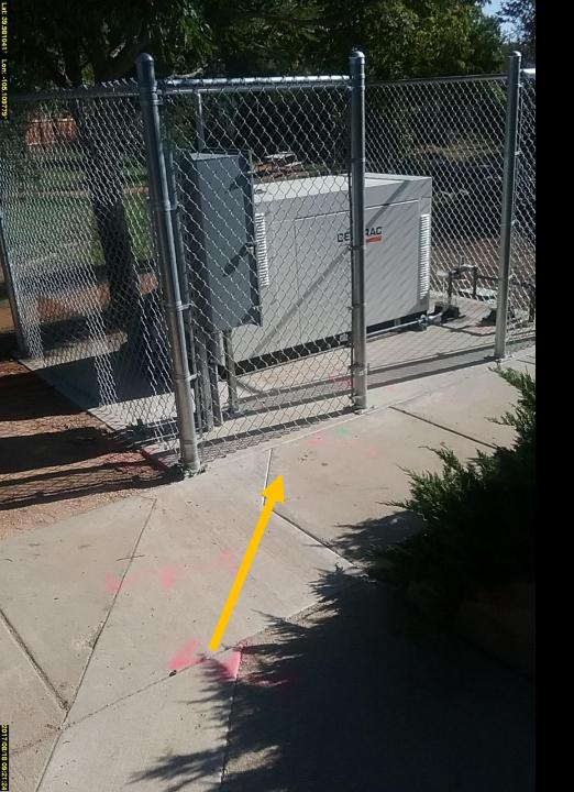
• Backup Generator. Several High voltage lines running to the building. If not properly identified and marked could result in serious injury if hit during excavation.
